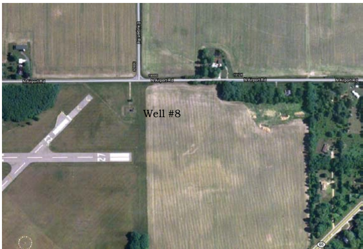
19. Aerial View of Well #8
